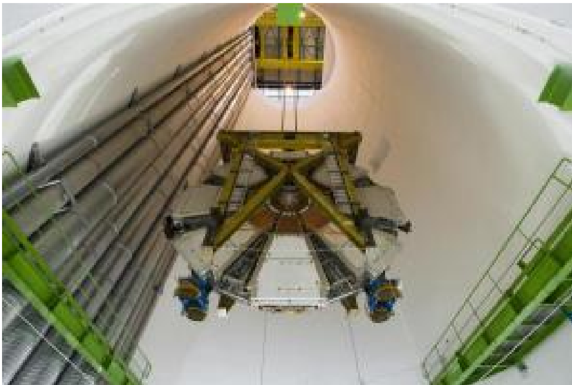
Lowering of the second ATLAS Muon small wheel. (Credit: Image courtesy of CERN)
